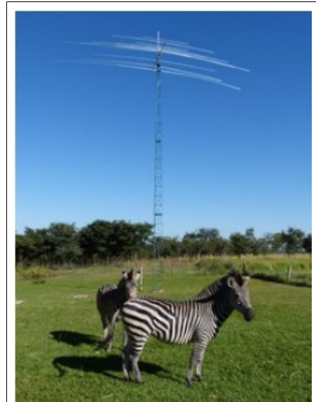
If you line up the zebras just right - do their stripes interact with the Yagi elements? This is a brand new Force 12 XR6 HF+6 Yagi installed at 9J2MM. Listen for the big new signal out of Zambia! (Photo from GØKSC)
