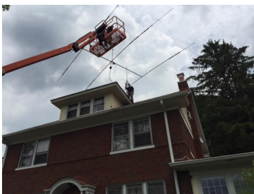
Cushman A3 Triband beam installation.
